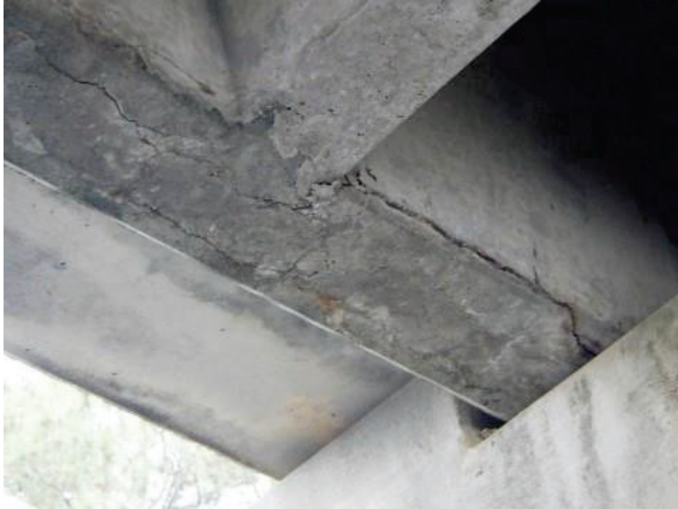
110 - Re Conc Opn Girder/Beam
