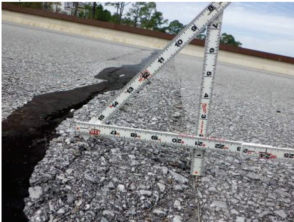
16 - Re Conc Top Flange (510 - Wearing Surfaces)
