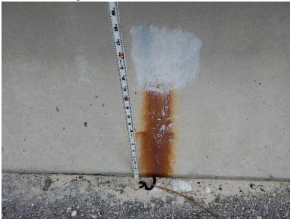
331 - Re Conc Bridge Railing
