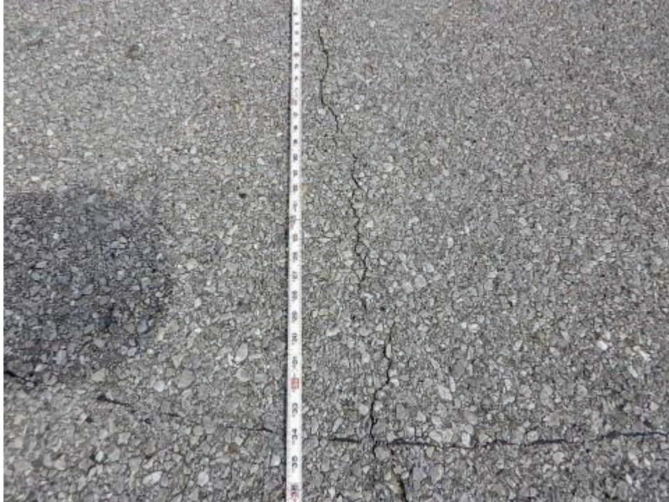
16 - Re Conc Top Flange (510 - Wearing Surfaces)
