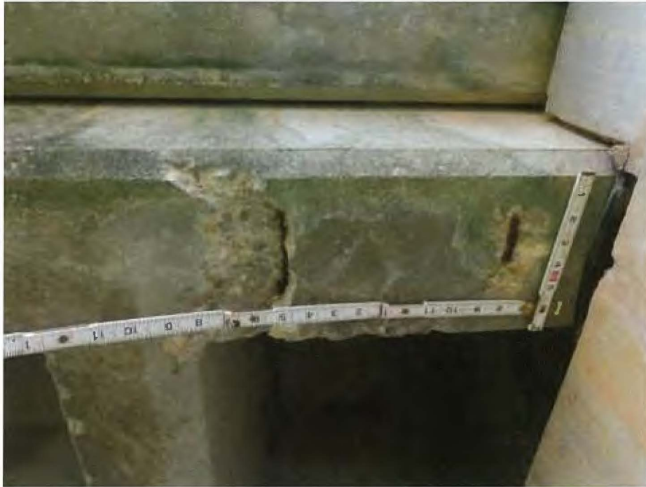
109 - Pre Opn Conc Girder/Beam
