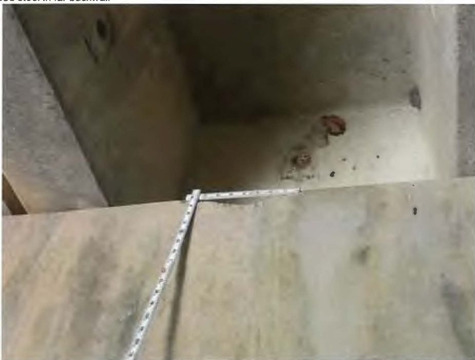
215 - Re Conc Abutment
