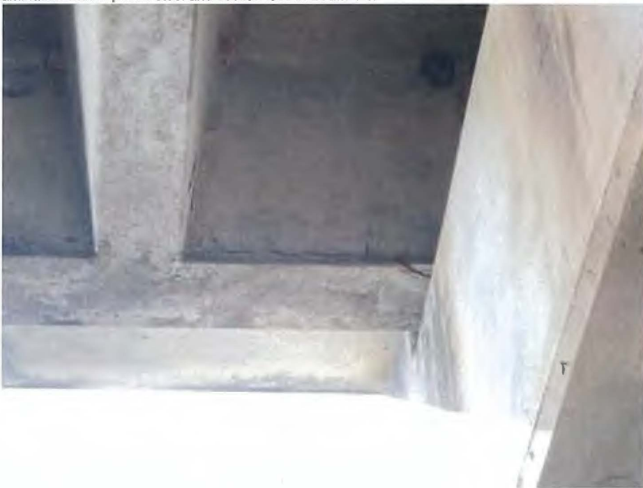
109 - Pre Opn Conc Girder/Beam
