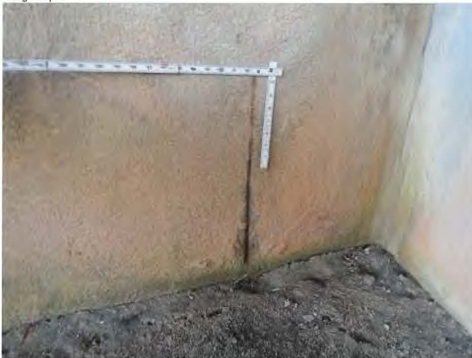
215 - Re Conc Abutment
