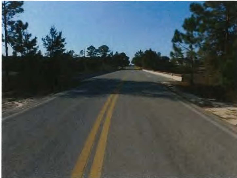
12 - Re Concrete Deck
