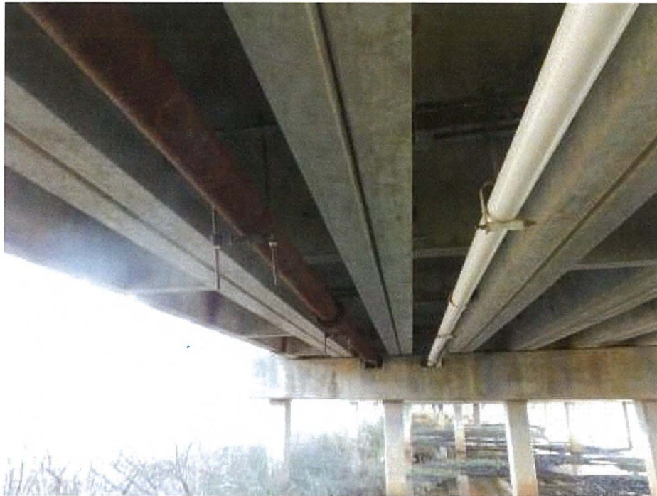
12 - Re Concrete Deck
