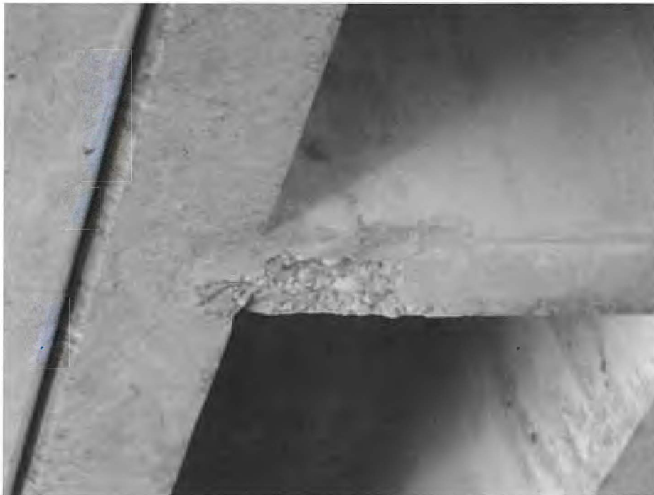
109 - Pre Opn Conc Girder/Beam
