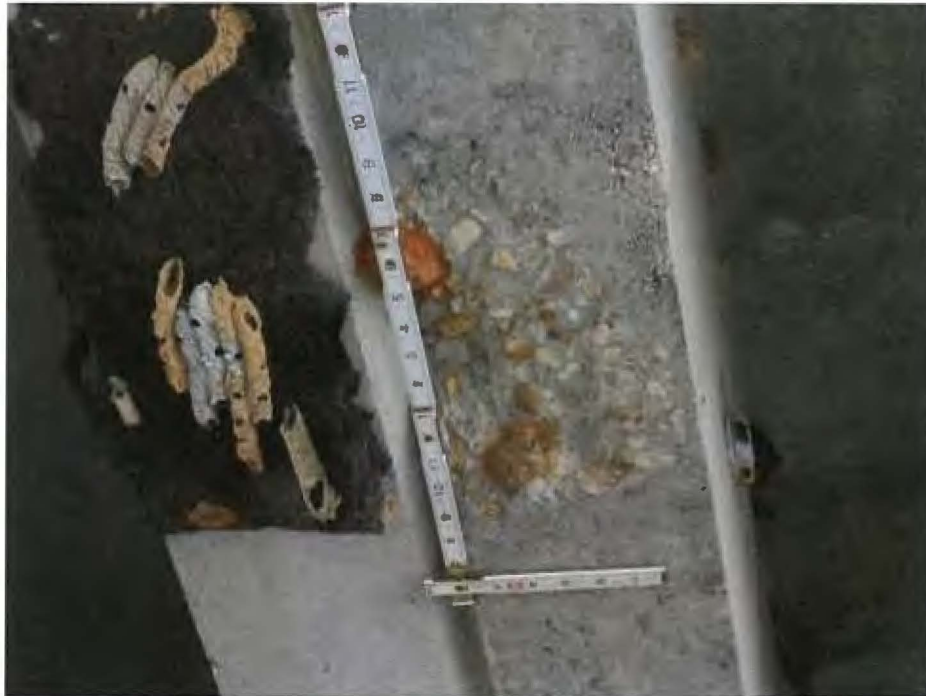
109 - Pre Opn Conc Girder/Beam
